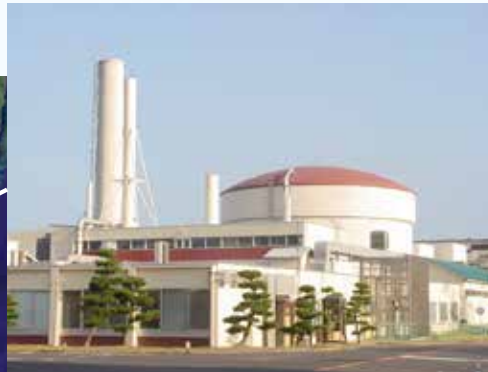
JRR-3@Japan Atomic Energy Agency (20MW Research Reactor)
